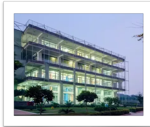
Lights ON during day hours
