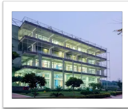
Lights ON during day hours
